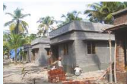
Construction of houses for the poor and needy
