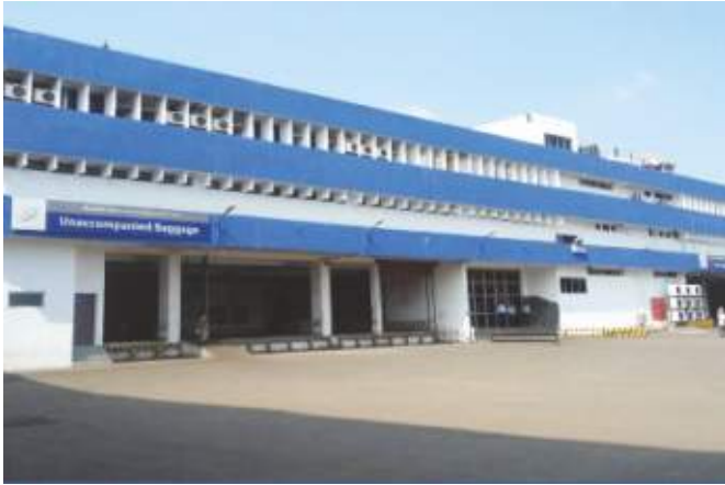
MIAL Air Cargo Complex Mumbai Project Value: INR 150 Million
