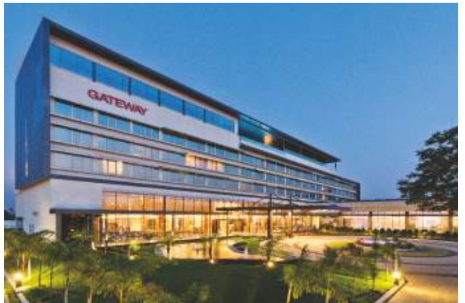
Taj Gateway Raipur Project Value: INR 25 Million
