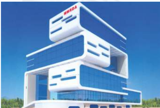
MMRDA BKC Mumbai Project Value: INR 190 Million
