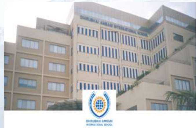
Reliance School Mumbai Project Value: INR 15 Million
