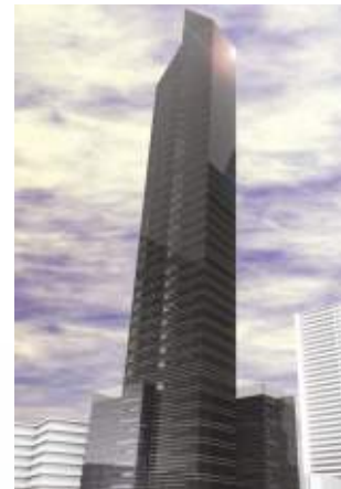
Lodha Washington House Mumbai Project Value: INR 65 Million
