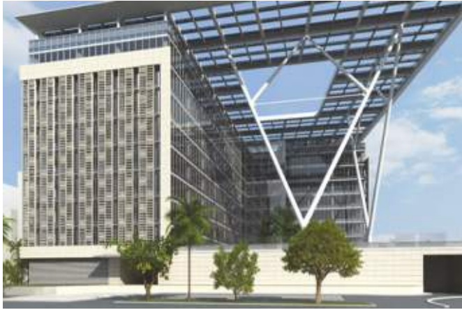
Reliance GHQ Mumbai Project Value: INR 120 Million
